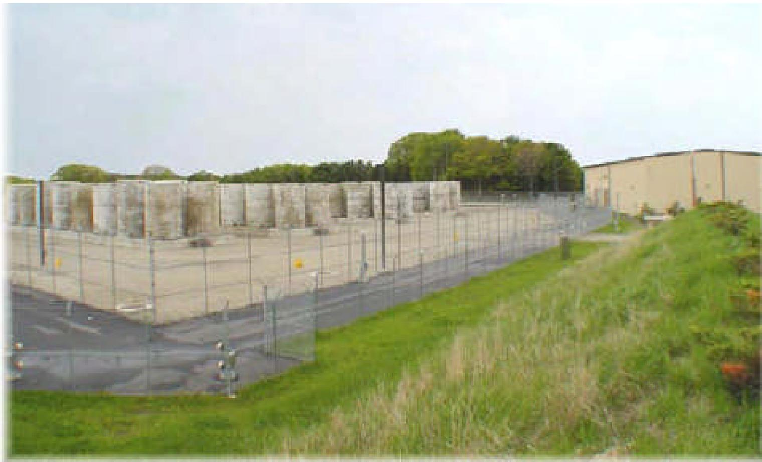
**Figure 9. Dry cask storage of spent fuel.** Two casks typically contain the equivalent of a year's spent fuel discharges from a 1000 MWe nuclear power plant. Comparison of the simplicity of interim spent fuel storage with the complexity of the huge reprocessing complex shown in Figure 6 makes it easier to understand the relatively low cost of interim storage.<sup>87</sup>
